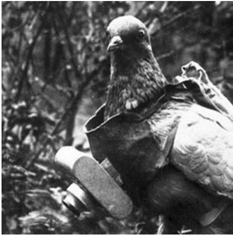
A pigeon with a special harness that allows it to hold a camera on its underside while flying
